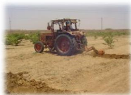
Figure 1c: Water Channeling Operation
